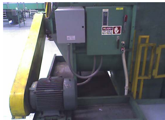
TYPICAL INSTALLATION AT SERVICE DISCONNECT
