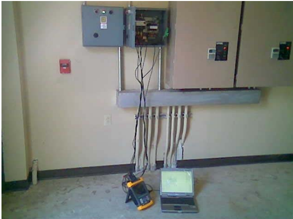
TYPICAL ASSESSMENT WITH FLUKE 434 AND LAPTOP
