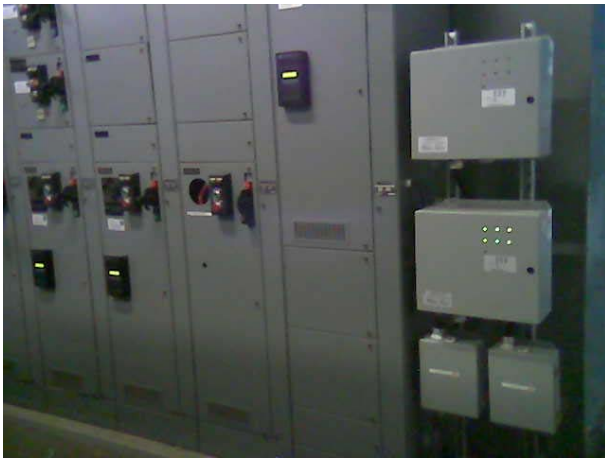
TYPICAL PANEL INSTALLATION FOR SOFT START APPLICATIONS
