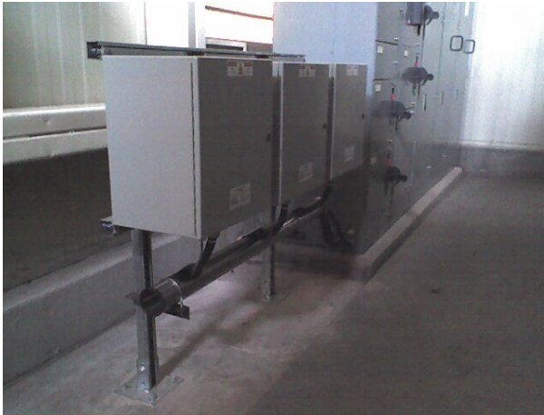
TYPICAL PANEL MOUNT INSTALLATION
