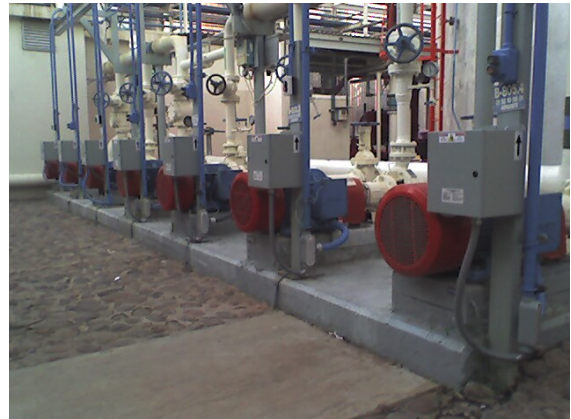
TYPICAL INSTALLATION AT MOTOR CONNECTION
